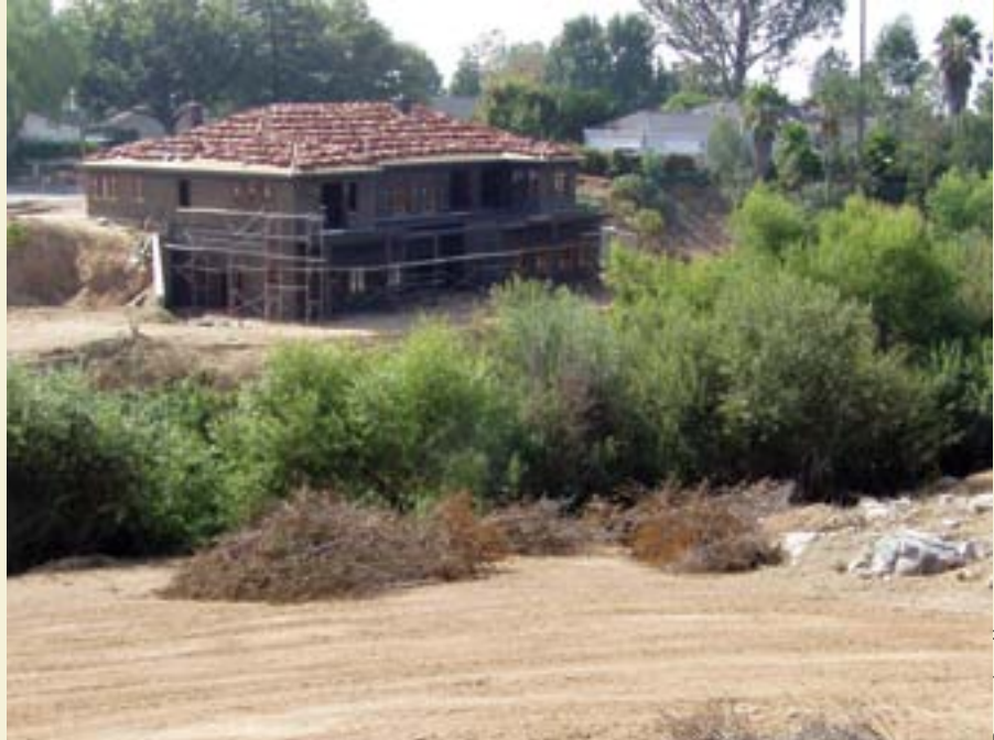
Encroachment too close to a waterway compromises its ability to function properly.
