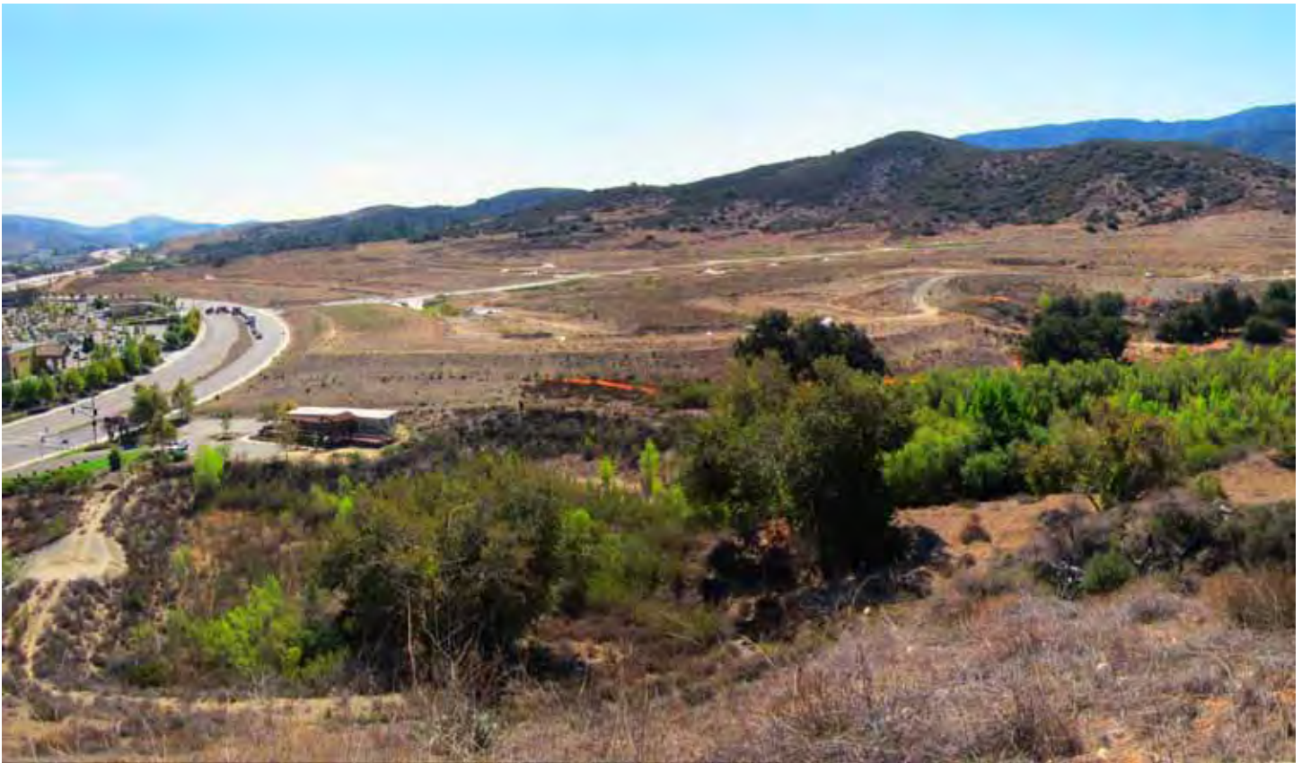
©2012-RIVERSIDE-CORONA RCD. ALL RIGHTS RESERVED PHOTO BY SHANI PLYNN View of the Field Office at Sycamore Creek Preserve.
