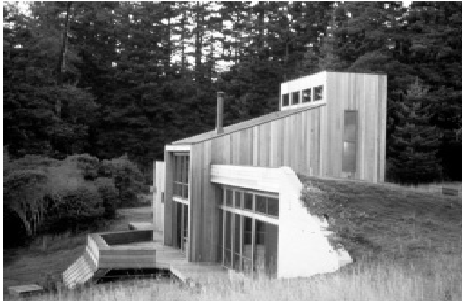
Design buildings to capitalize on site conditions. This house was designed to harvest solar radiation and to use the earth as an insulator.
