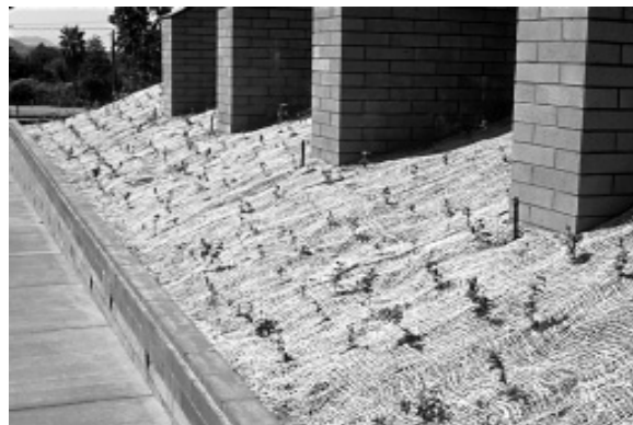
Jute netting holds the soil in place until new plants become established. Plant roots will anchor the soil, while the tops of plants will intercept the force of pounding raindrops. When left on the soil surface, dead plant debris acts as a mulch.
